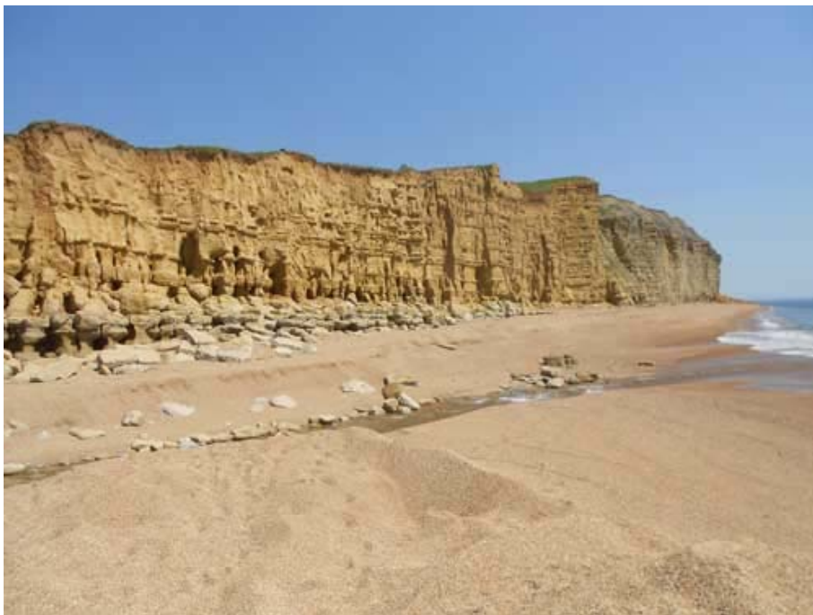
The yellow sandstone cliffs between Freshwater Bay and Hive Beach that are shaped by erosion processes, including landslides. Taken 25 July 2012.
