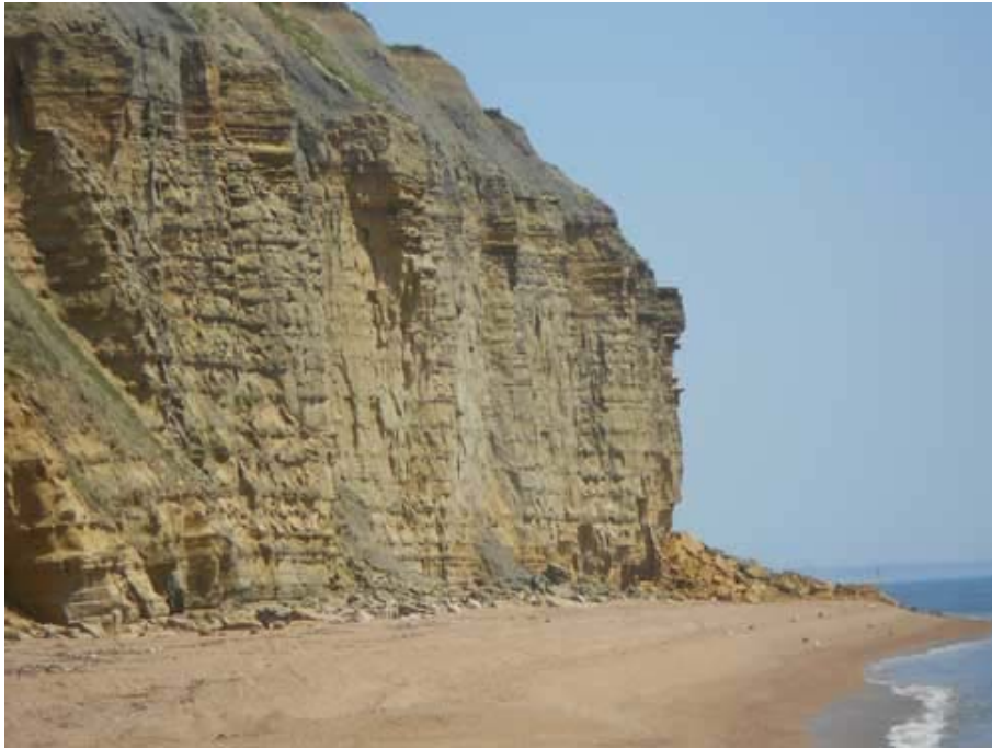
Eroding piles of rock debris along the base of the Jurassic sandstone cliffs at Burton Bradstock are telling signs of continual erosion by landslides. Taken 25 July 2012.
