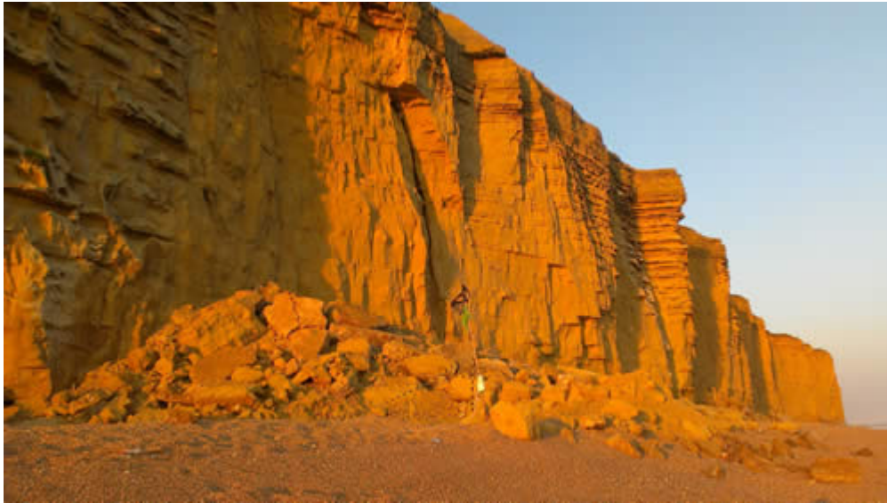
The Burton Bradstock rock fall landslide of 24 July 2012.
