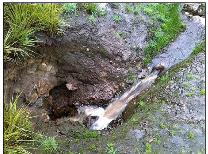
Photo 4: Water drains from Pwll-y-Felin via a discrete conduit in the base of the doline. The low-permeability glacial till deposits that line the doline can also be observed to a thickness of at least 1.5m. (BGS© NERC.)
