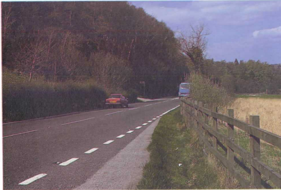
Plate 14. A roadside verge showing typical low vegetation maintained by a regime of spraying and cutting
