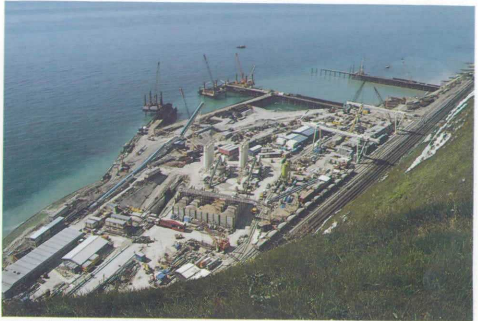
Plate 1. View of Channel Tunnel platform from Shakespeare Cliff
