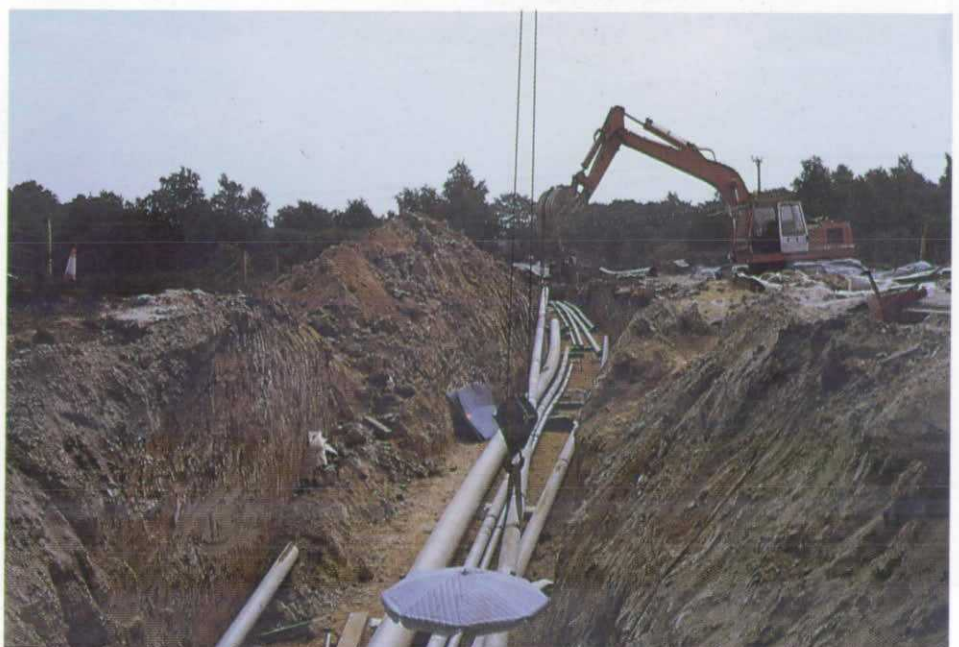
Plate 3. Stoborough Heath. Multiple pipelines being assembled in trench deepened to pass under a road
