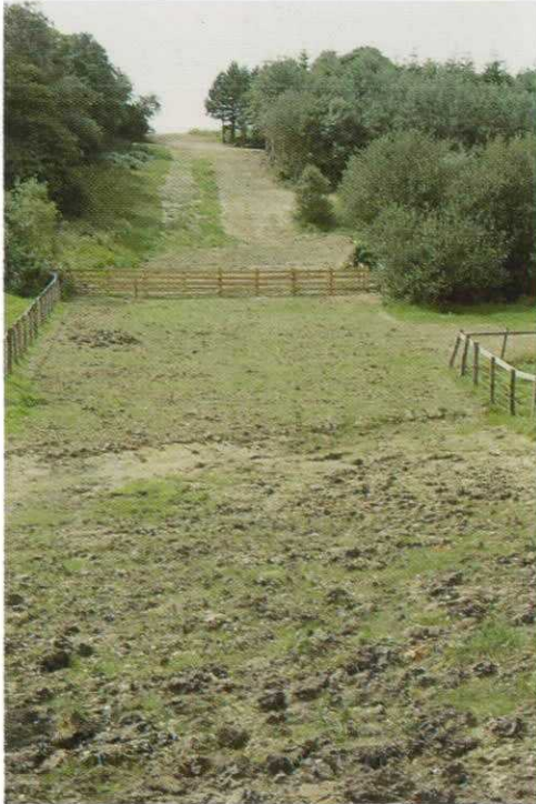
Plate 4 Chale Wood. Restored pipeline route with first stages of recolonisation taking place
