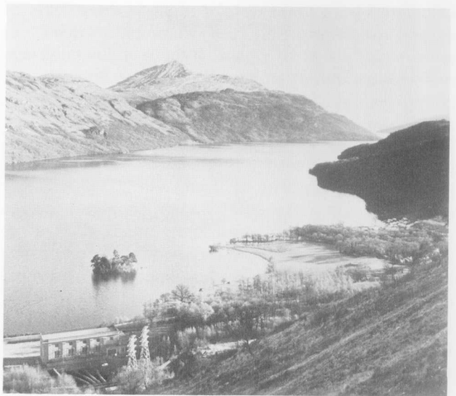
Plate 1 Lamprey studies are being carried out at Loch Lomond, seen here looking south-east, across Sloy hydro-electric power station, towards Ben Lomond (Photograph S V Mills)
