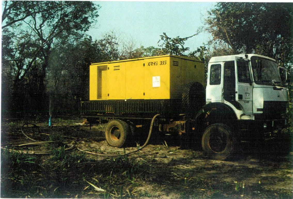
Plate 6 Cleaning completed borehole using compressed air at Nyambekyere
