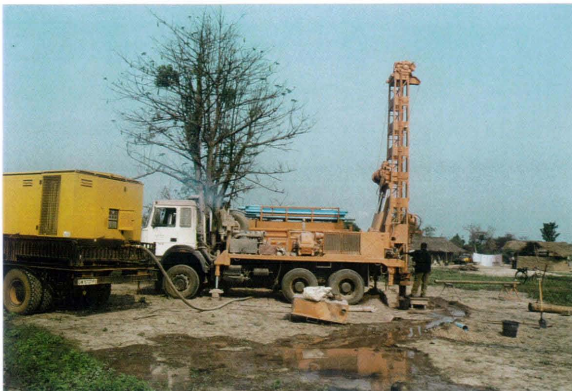
Plate 1 Geomechanik drilling rig mounted upon a 6x4 truck chassis with Atlas Copco compressor mounted on a 4x4 truck chassis at Asanyansu borehole drilling site
