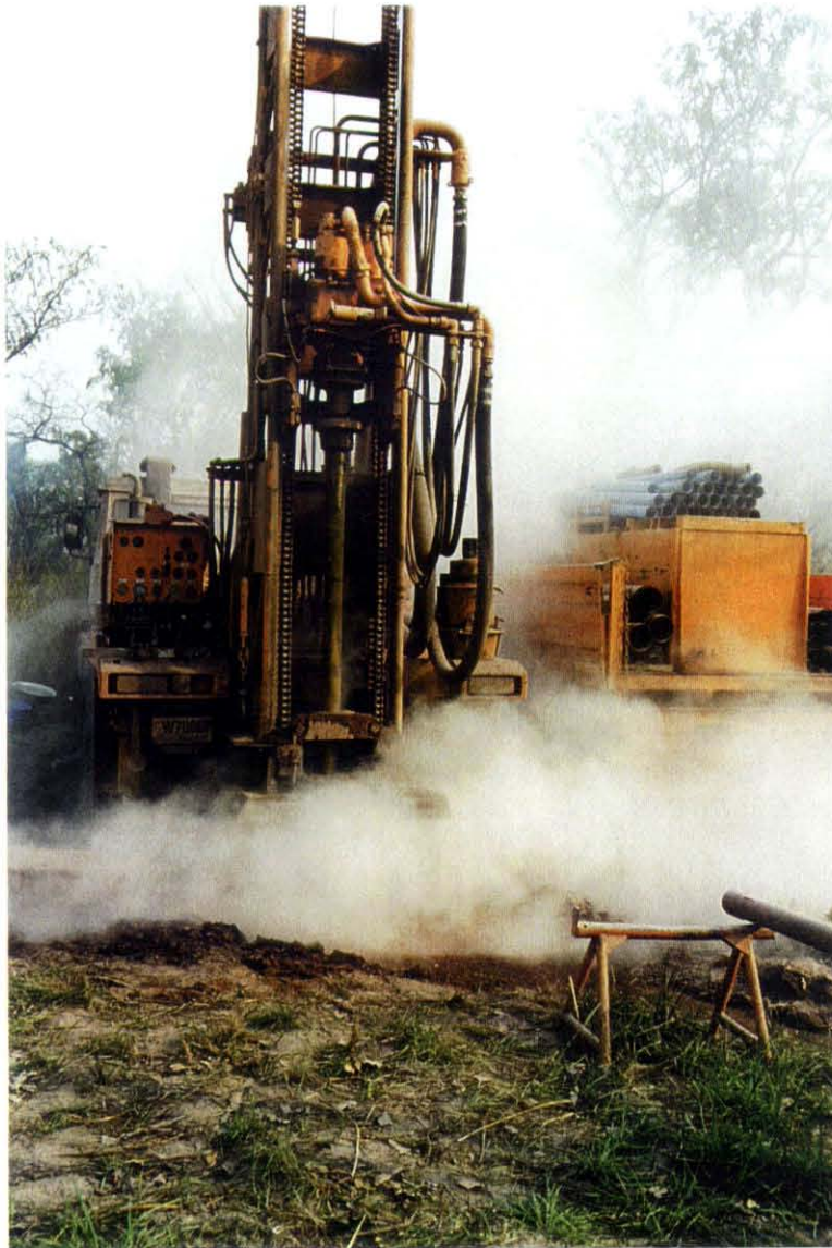
Plate 3 Dusty conditions when drilling with compressed air at Nsareye "A".
