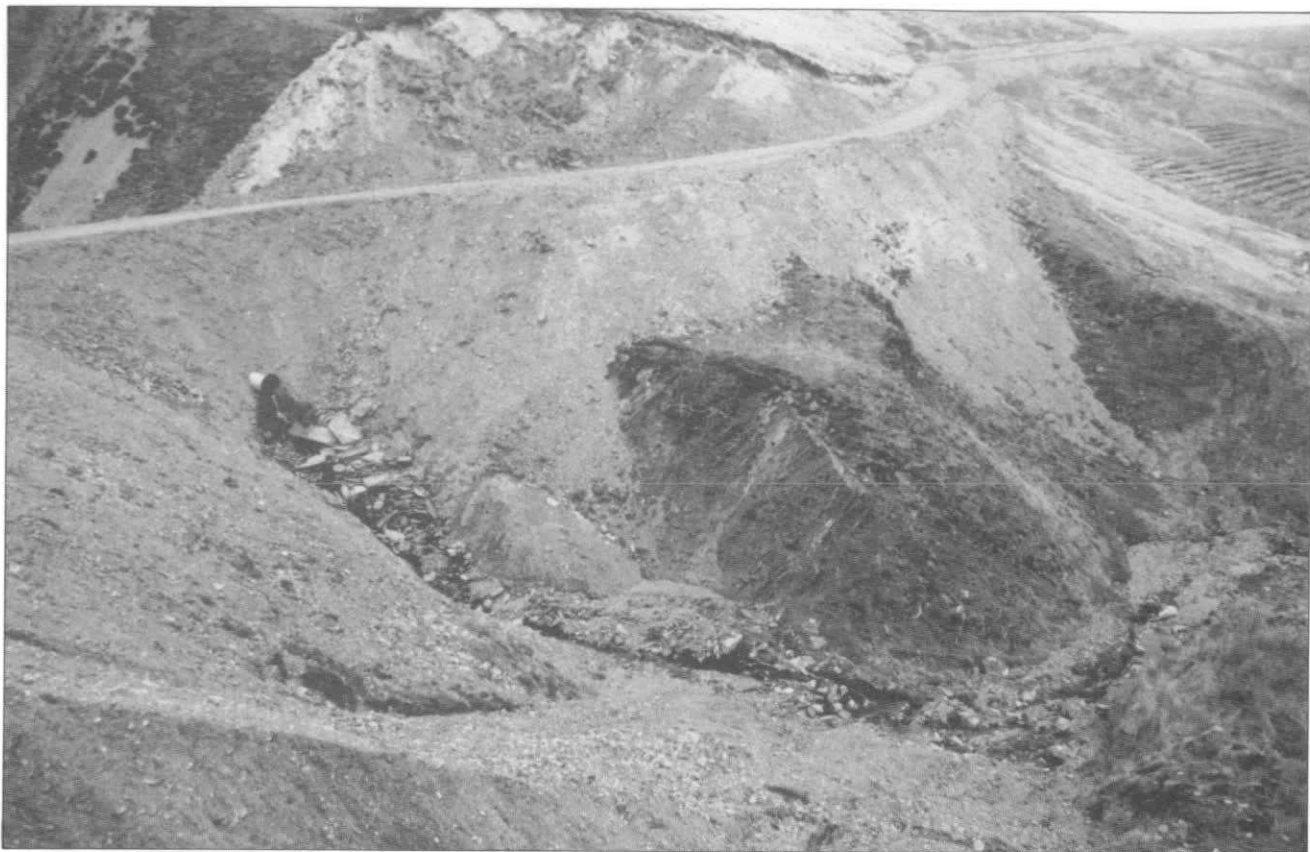
Plate 4. Loose gravels, exposed on steep road embankments, are readily transported by gravity and gully erosion into the stream channel. Afon Cwm catchment, Llanbrynmair (Photograph G J L Leeks)
