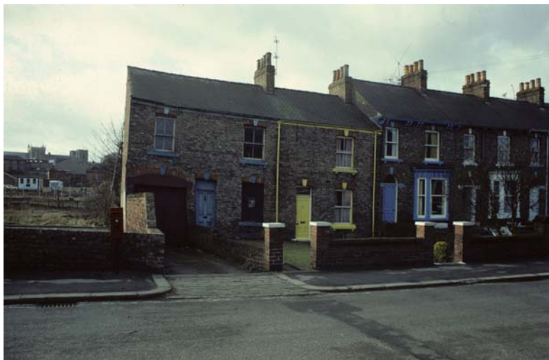
Figure 3. Sagging building damage Category 5 caused by gypsum dissolution and associated settlement on peat deposits, Princess Road, Ripon (Cooper, 1998).
