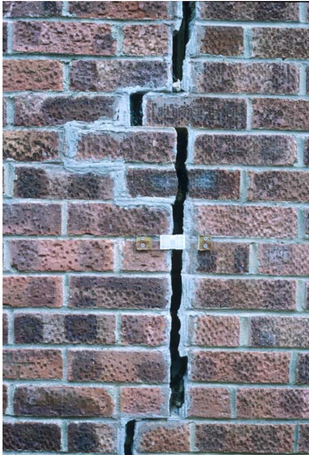
Figure 6. 18 mm crack in wall of house at Hutton Conyers near Ripon, damage caused by subsidence at side of large doline formed by the dissolution of gypsum. Category 4 damage formed by loss of support and rotation of the floor slab.
