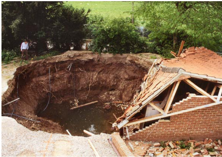
Figure 2. Category 7 building damage at Ure Bank Terrace, Ripon. The damage here has been caused by gypsum dissolution and collapse with loss of support under most of the building (Cooper, 1998).
