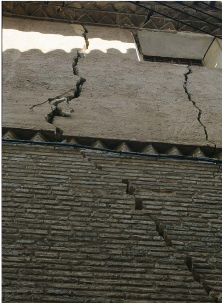
Figure 5. Cracks in historic building of Colegiata Sta. María La Mayor in Calatayud, Spain, here the cracks are up to 30 mm wide, others on the building are larger and the degree of damage merits a Category 5 classification, (Gutiérrez and Cooper, 2002).
