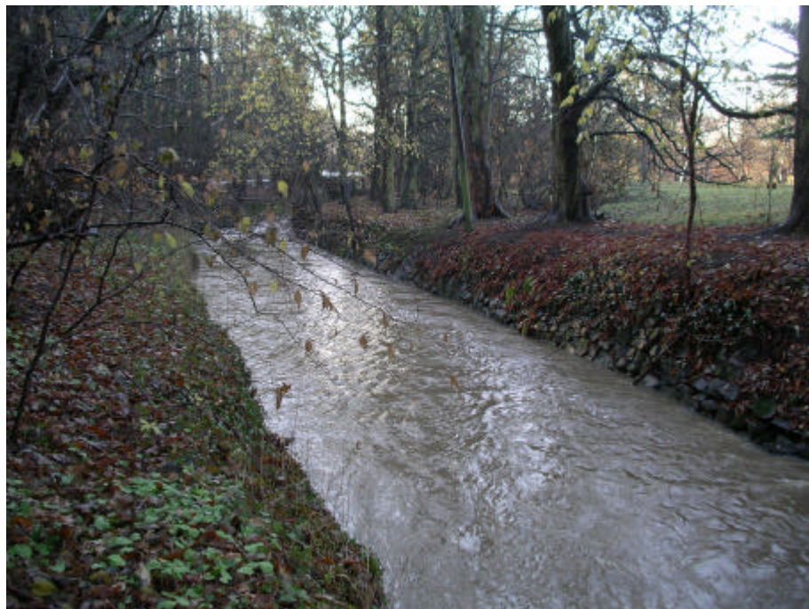
Figure 2 Bank reinforcement and resectioning near the RBS headquarters (site 2)
