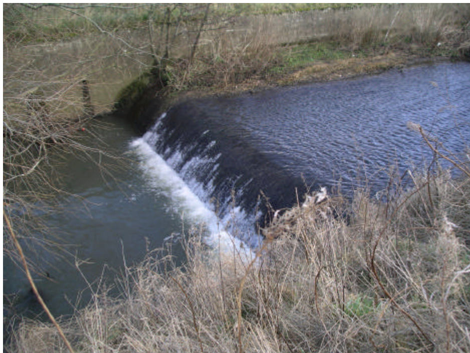
Figure 3 Weir at Turnhouse (near Edinburgh airport)
