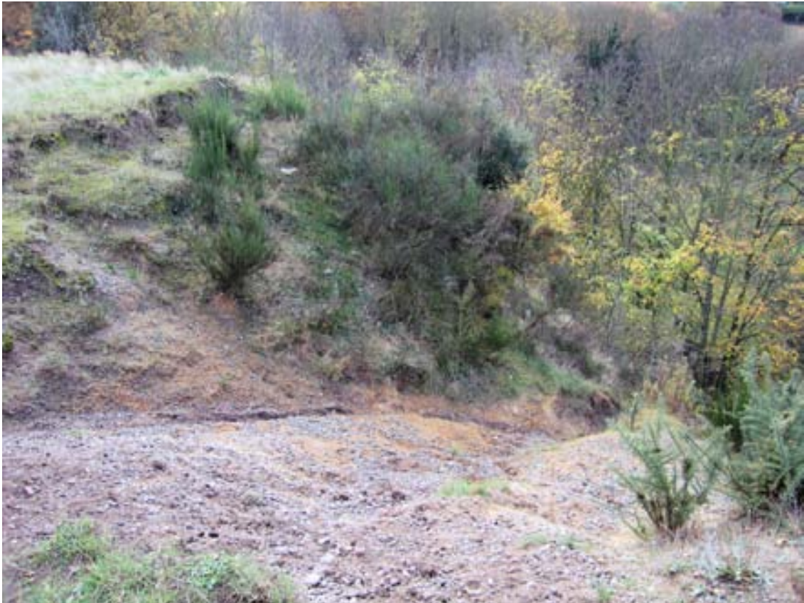
Slumped material viewed from top of site
