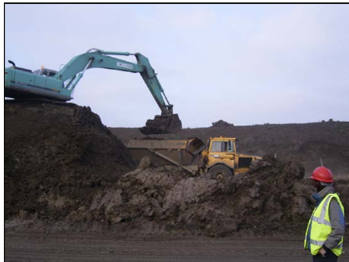
Figure 10: Sampling from a spoil heap of unweathered London Clay at Roxwell landfill site
