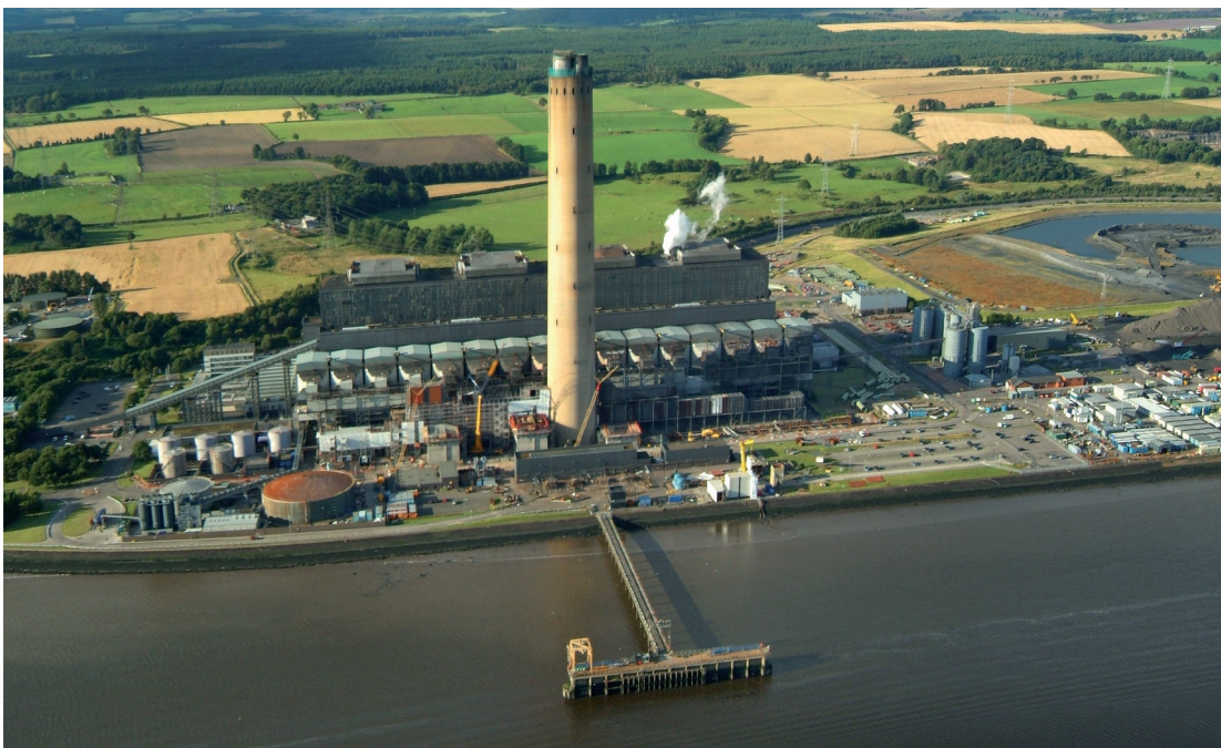
Figure 1.2 Image courtesy of Scottish Power. Longannet coal fired power plant, Firth of Forth
