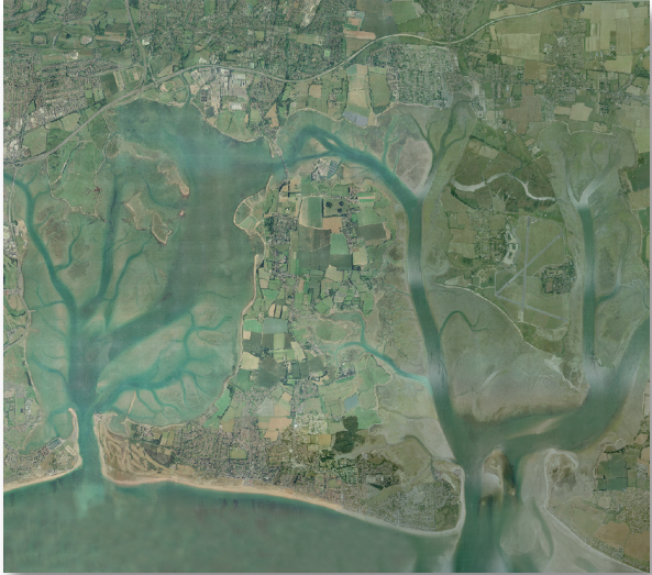
Figure 33 Aerial view of Langstone and Chichester harbour © UKP/ Getmapping Licence No. UKP2006/01.
