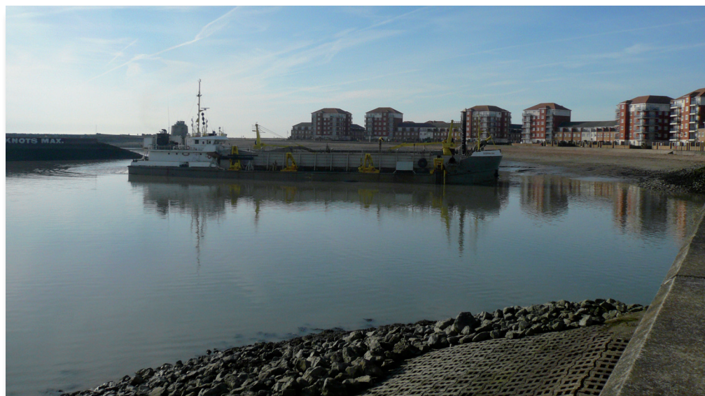
Figure 15 Maintenance dredging at Sovereign Harbour, Eastbourne, March 2010. Material disposed at Eastbourne site.
