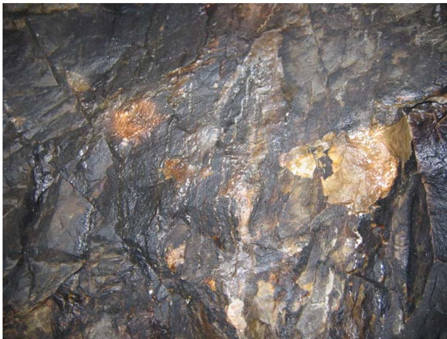
Figure 6 Groundwater seepages along fractures
