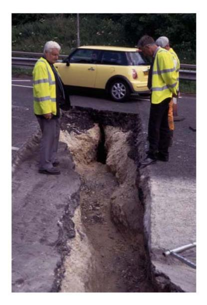
Figure 5. Fissure exposed beneath the near-side lane of the north-bound carriageway of the A690, 20 June 2003. Walls of solid dolomitic limestone and an open fissure beneath the tarmac can be clearly seen.
