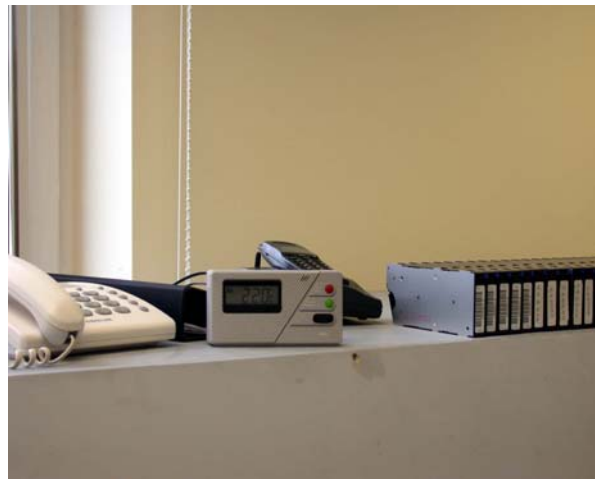
Plate 5: SNS Server Room (Near A/C Unit)
